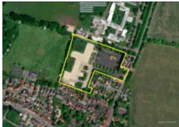
Site of the former Council Offices, Crowmarsh Gifford
