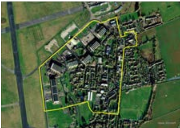
Brownfield land at Dalton Barracks
